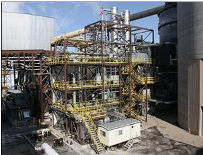
Alstom and the Electric Power Research Institute have opened this plant in Wisconsin to test the use of chilled ammonia to capture CO2 from power plant emissions. Photo courtesy of Electric Power Research Institute.
